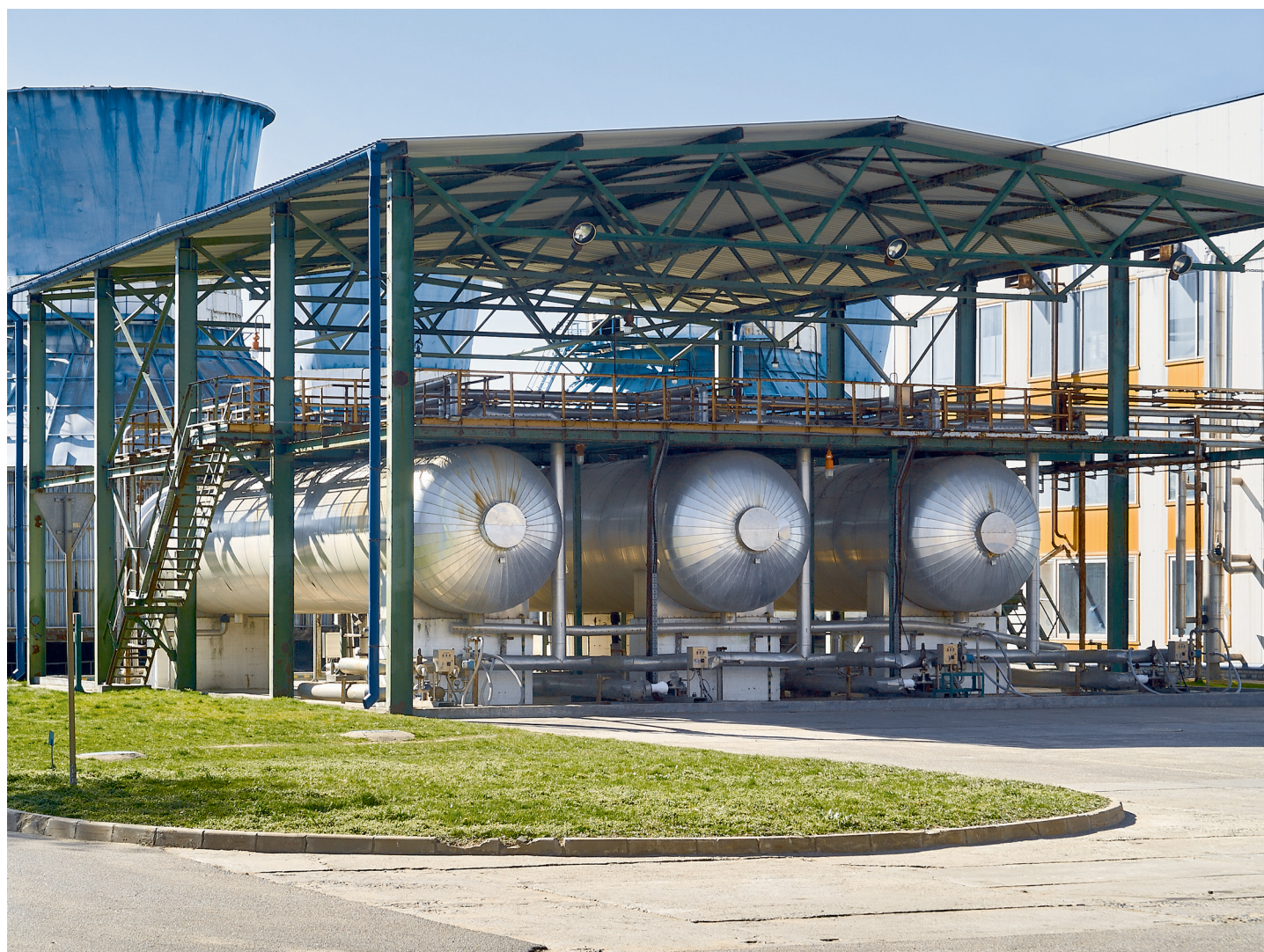
Cryogenic liquid CO 2 storage tanks
