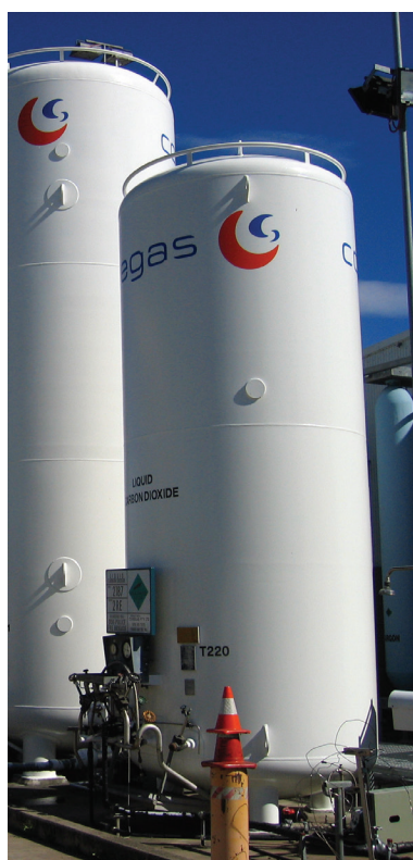
Coregas bulk CO 2 tank
