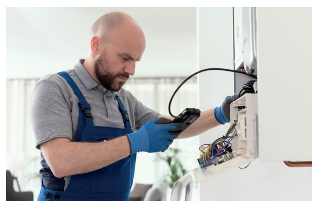
Testing flue gases from a domestic boiler
