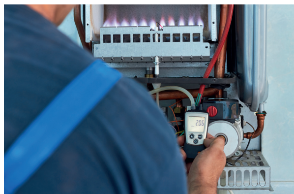
Flue gas testing on a boiler
