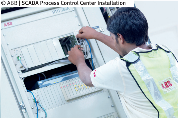
© ABB | SCADA Process Control Center Installation
