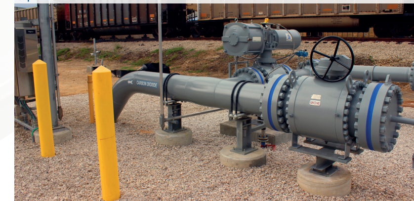
© NRG Energy Inc | Petra-Nova's captured carbon dioxide pipeline
