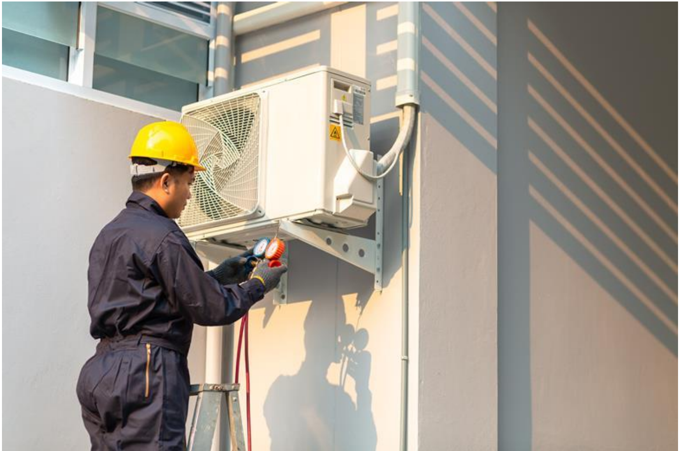
HVAC refrigeration F-Gas system maintenance
