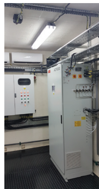
Copyright ABB - ACF5000 FTIR CEMS installation
