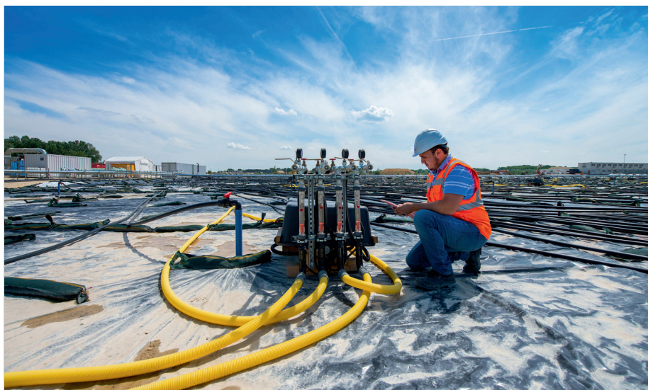
Photo: AUDI AG IN-Campus Environmental remediation of legacy refinery at Ingolstadt - air sparging unit
