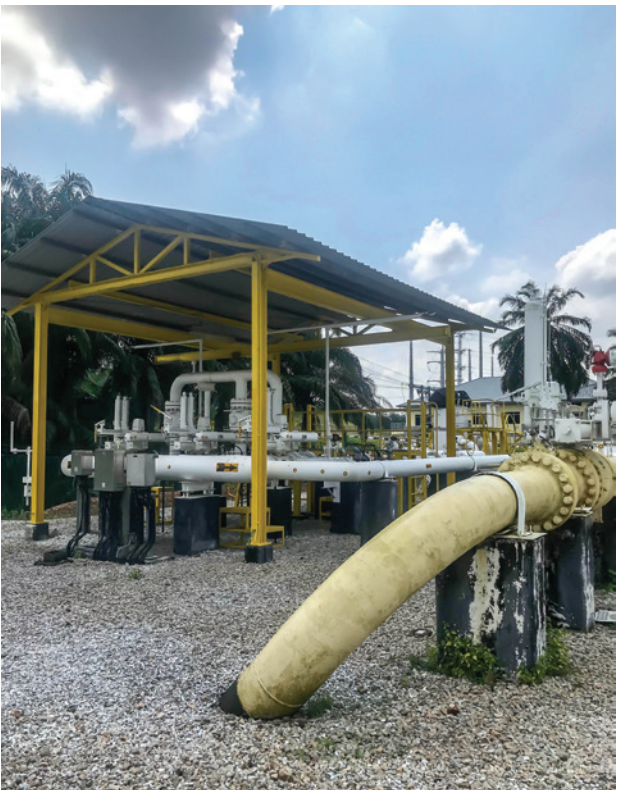
Gas pipeline flow and purity monitoring station
