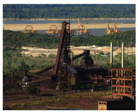
Direct Reduced Iron (DRI) is produced by passing hot reducing gases such as hydrogen, natural gas, or syngas over iron ore. DRI can be produced as briquettes which are sometimes referred to as hot briquetted iron (HBI), pellets, or lumps. HBI and DRI are likely to become major international cargoes as 'green steel' made from green hydrogen becomes more popular.
