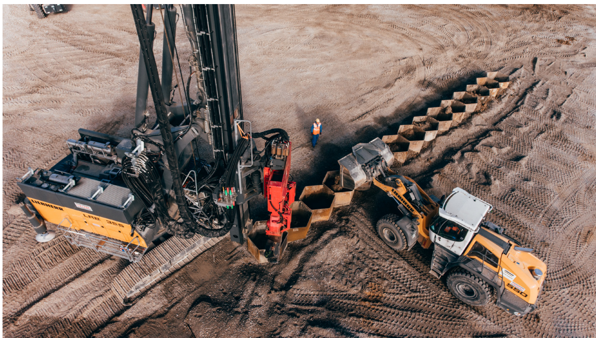
Copyright ZÜBLIN Umwelttechnik GmbH, Pile driving machine to enable deep soil excavation for washing
