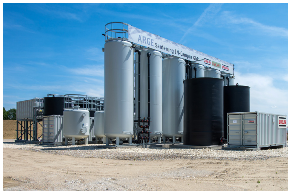
Copyright ZÜBLIN Umwelttechnik GmbH, Groundwater purification plant
