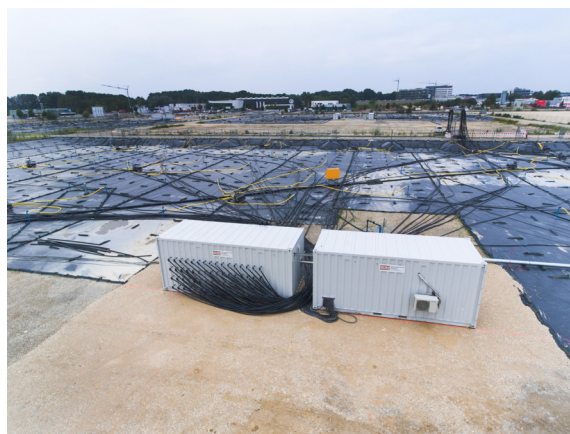
Copyright ZÜBLIN Umwelttechnik GmbH, Air sparging equipment is used to release lighter hydrocarbons for incineration or catalytic destruction
