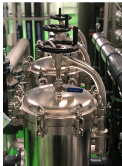
Activated carbon for removal of chlorine and organic molecules
