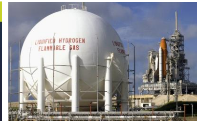
Liquid hydrogen storage at Cape Canaveral
