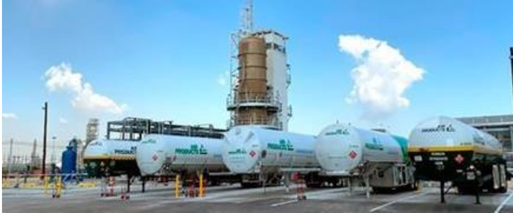
World scale hydrogen liquefaction in USA, 30 tonnes per day, Image: Chart Industries
