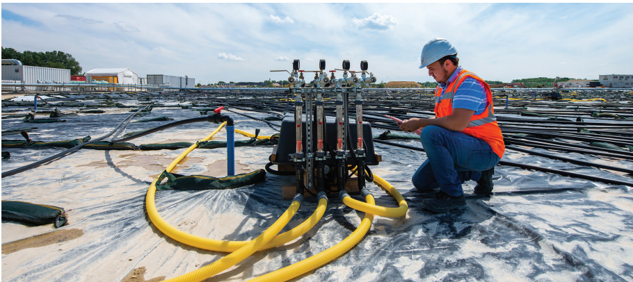
Copyright AUDI AG IN-Campus Environmental remediation of legacy refinery at Ingolstadt - air sparging unit
